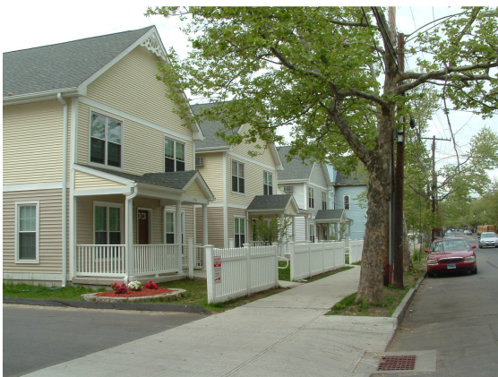
Typical street front building
