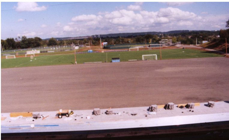
Field rough graded, geotextile fabric installed and stone drainage layer underway.
