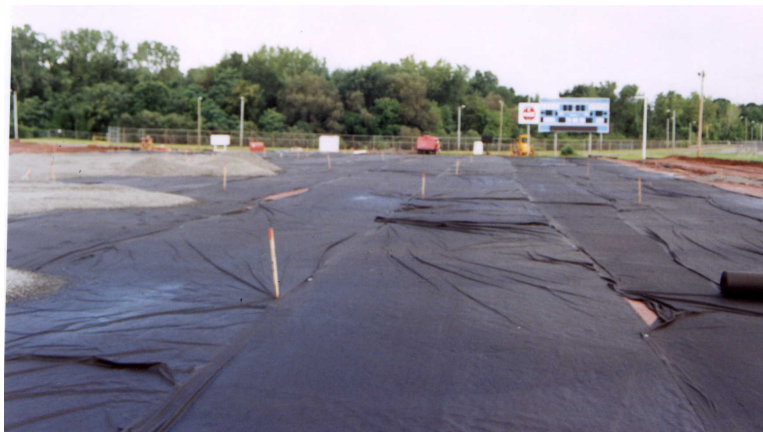
Field rough graded, geotextile fabric installed and stone drainage layer underway.
